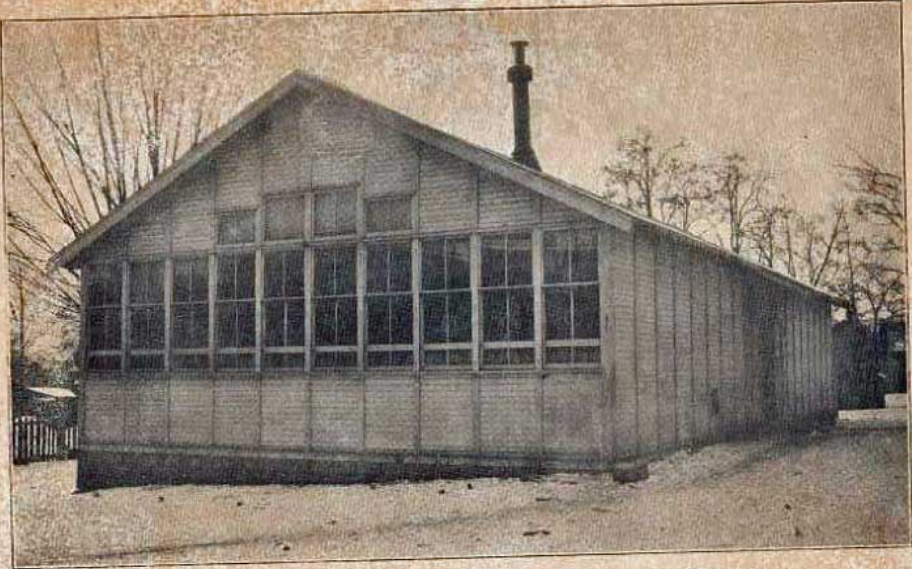
There is no effort to satisfy the appeal for beauty in the portable school building. It is a matter of direct utility with the added feature of saving the money of the taxpayer. The astonishing low cost is indicated in the fact that $2,908.32 has afforded class accommodations for children numbering between eighty and one hundred.
